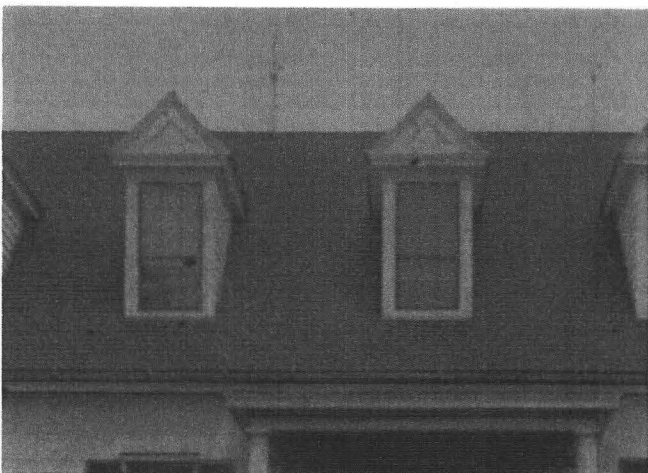
Figure 1.10 After the early-twentieth-century remodeling, the dormers exhibit a taller pediment and steeper pitch.
